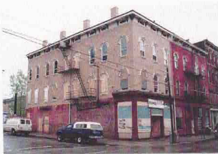
(18) Northwest Facade in Progress
