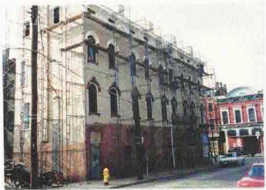
(14) Northeast Facade in Progress
