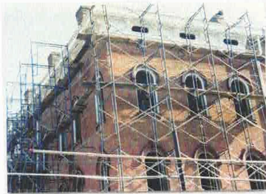
(13) West Facade in Progress
