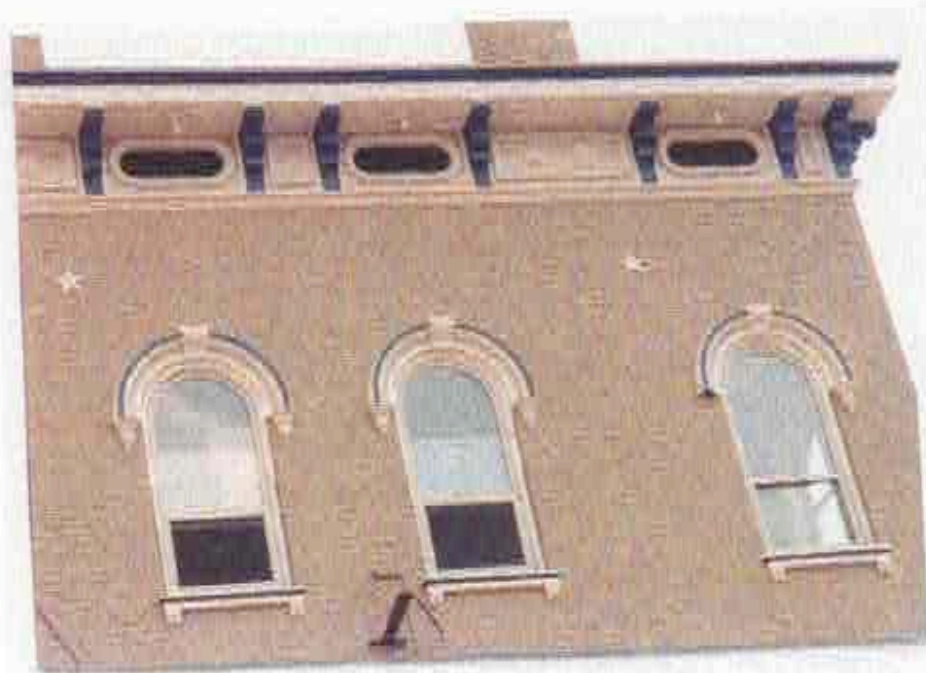
(17) Facade Cornice Detail Finished
