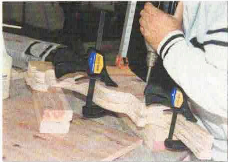
(08) Cornice Detail Rebuild
