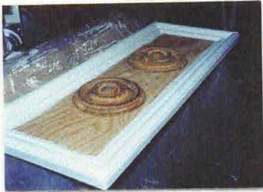
(11) Cornice Panel Repair
