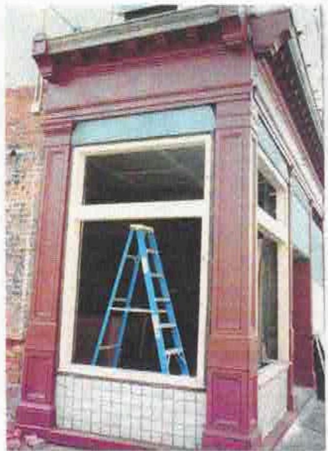
(16) North Facade Storefront
