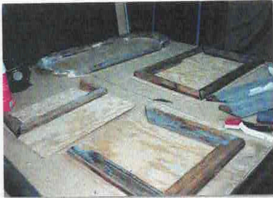
(07) Cornice Detail Repair
