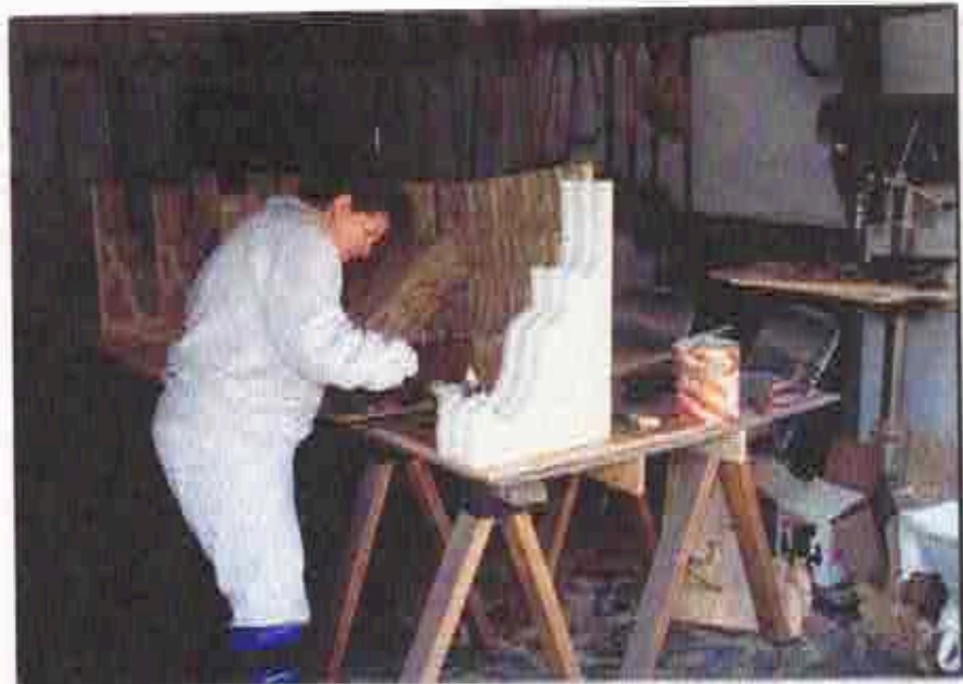
(12) Cornice Bracket Repair
